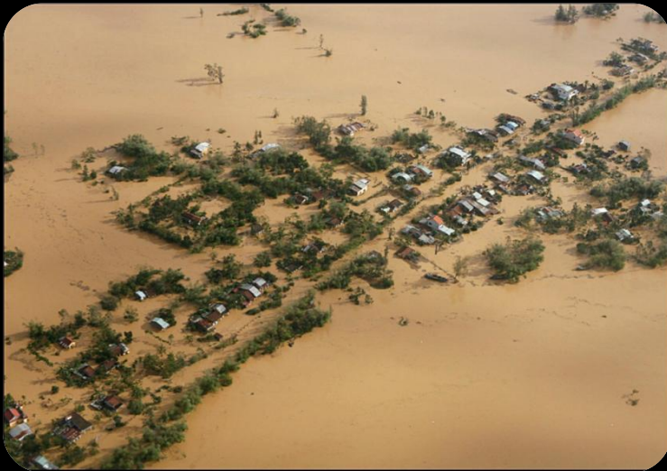
Recurring infrastructure damage productivity
